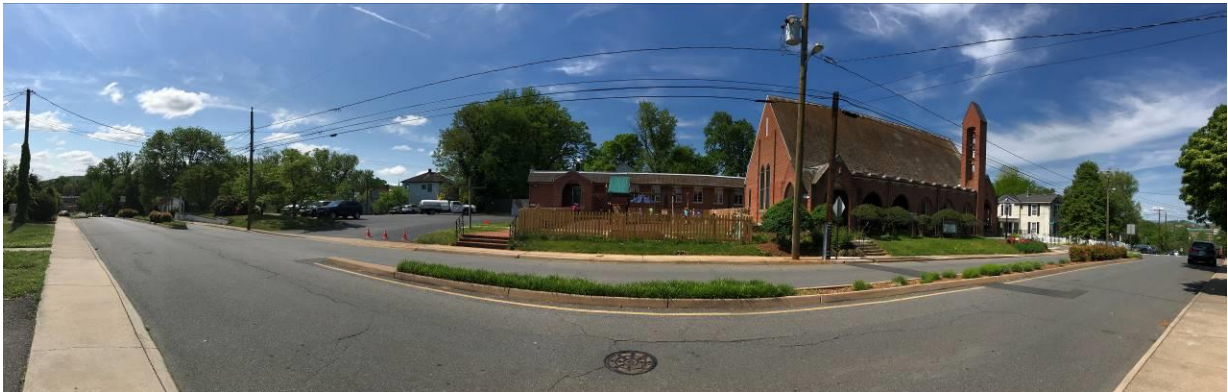
Photograph 1 – Elevation of Subject Property looking southward across Hinton Avenue
