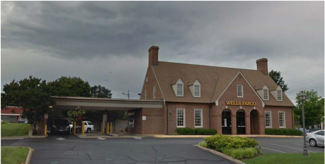
Existing structure and drive through canopy – SOURCE: Google Street View
