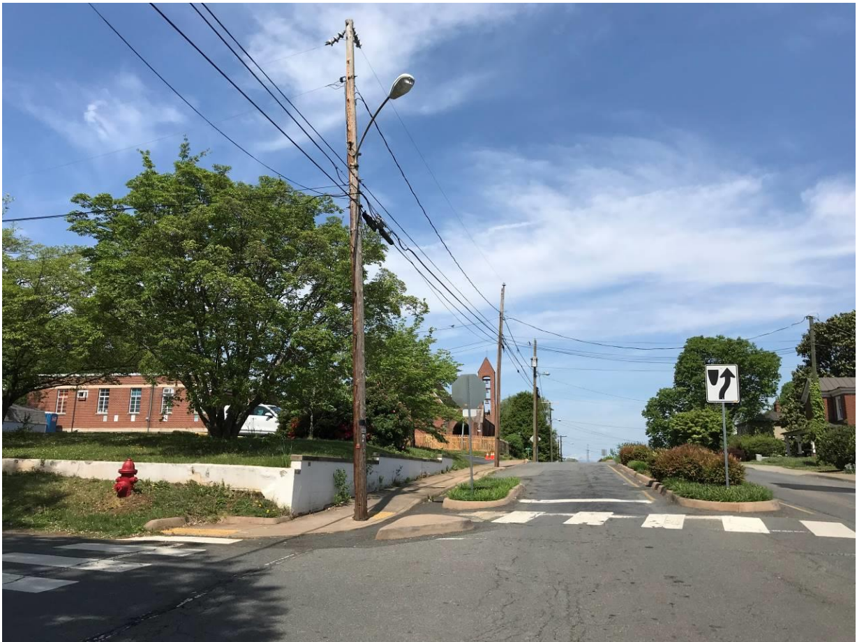
Photograph 2 – Looking at Existing retaining wall at the corner of Hinton Avenue and Rialto St.
