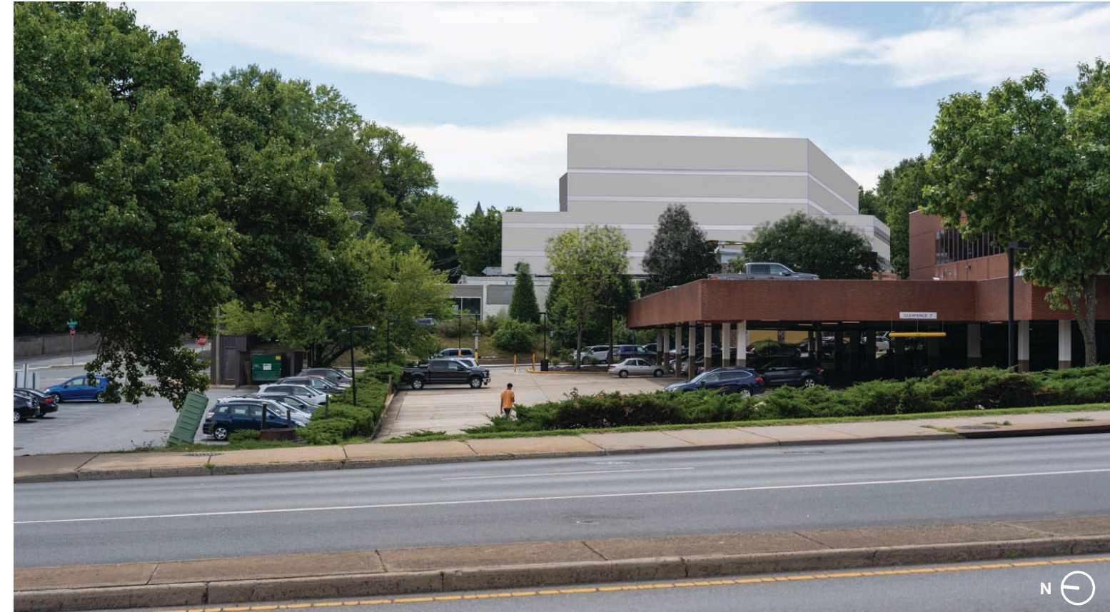
VIEW WEST ACROSS RIDGE MCINTIRE - BY RIGHT
