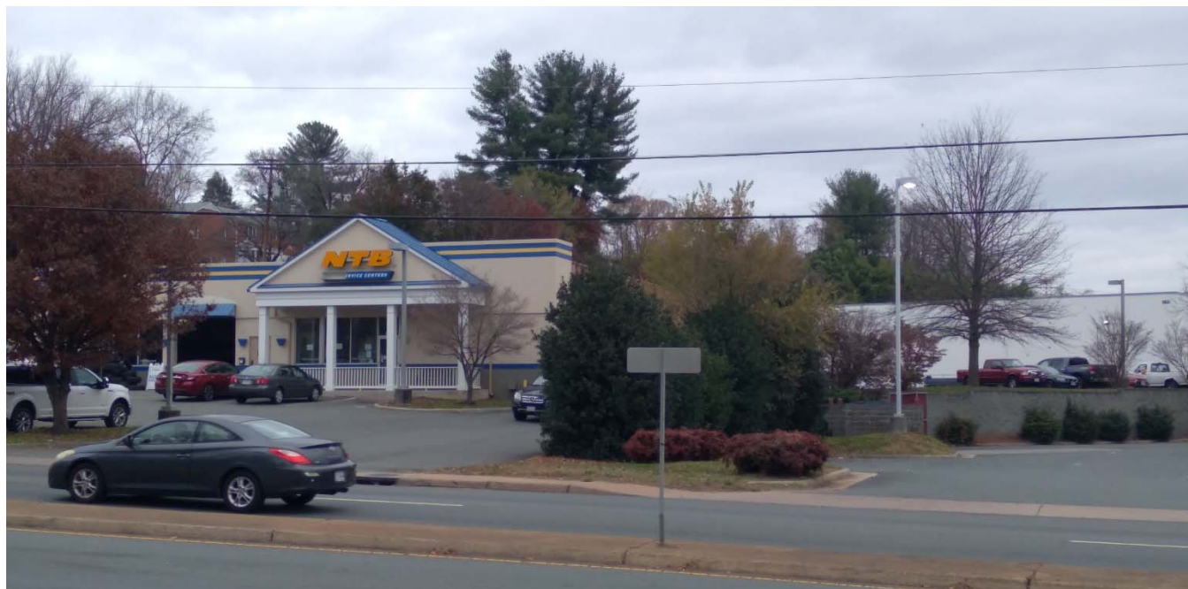
1321 LONG ST – NTB SERVICE CENTER
