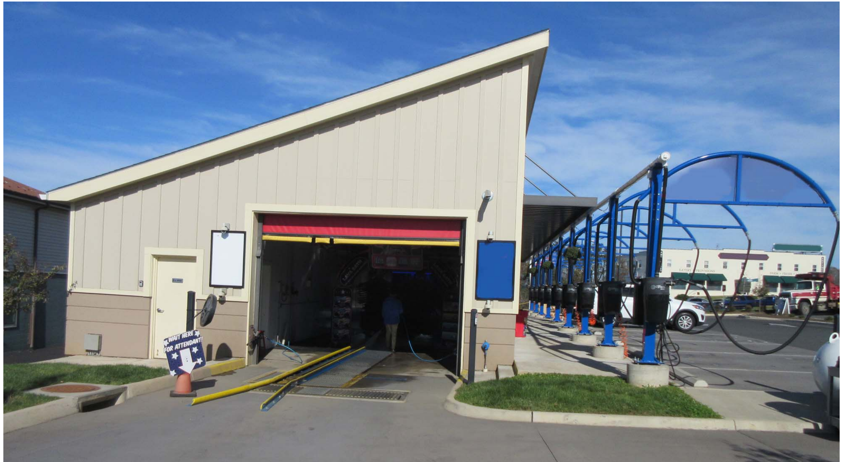
ELEVATION FACING ENTRANCE CORRIDOR
