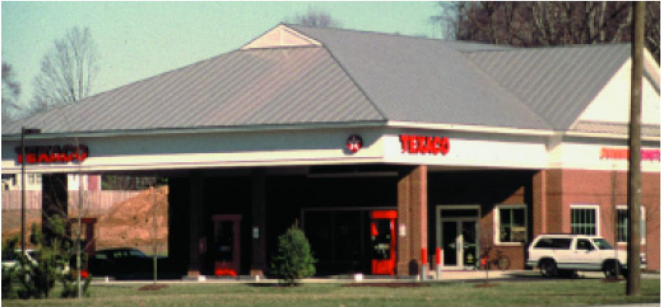
This gasoline canopy is integrated into the roof of the building and creates a more unified design than would a separate element.
