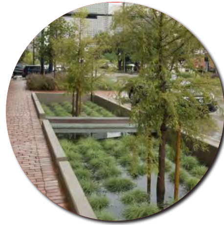
STORMWATER CONCEPT: MICRO-BIOFILTERS ALONG OBSERVATORY AVE.; NATIVE PLANTING AND WEIR WALLS/ TIERS TO SLOW THE MOVEMENT OF WATER
