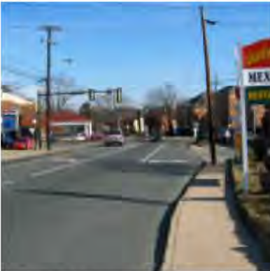
Sub-Area B: Lewis Street to Maury Avenue
