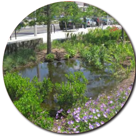
STORMWATER CONCEPT: MICRO-BIOFILTERS ALONG OBSERVATORY AVE.; NATIVE PLANTING AND WEIR WALLS/ TIERS TO SLOW THE MOVEMENT OF WATER
