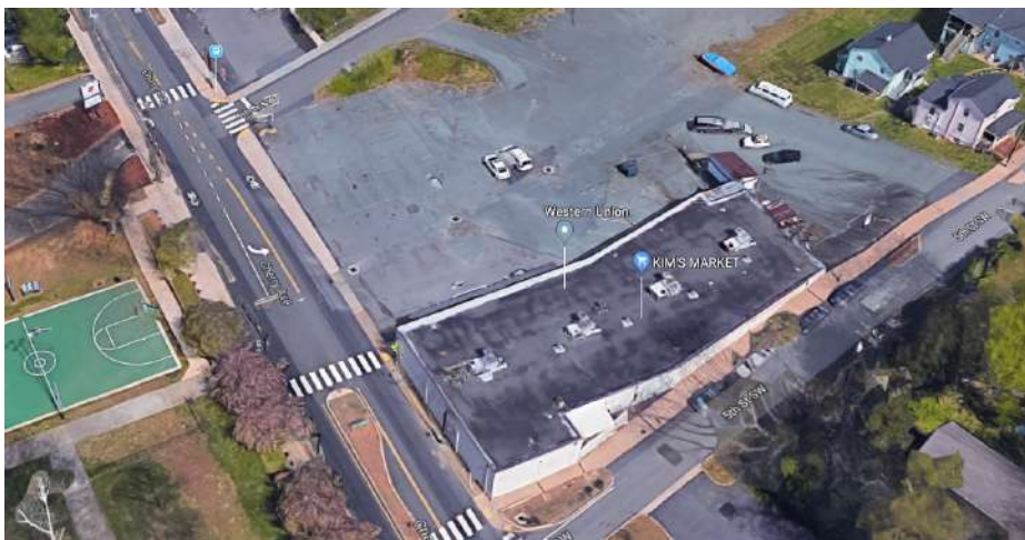
Aerial shot of existing Kim’s Market at Site 2 facing west down Cherry Street.
