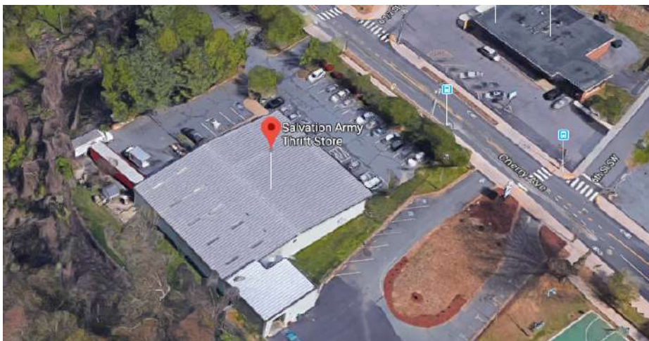
Aerial view of existing conditions at Site 4 looking north toward Cherry Avenue.
