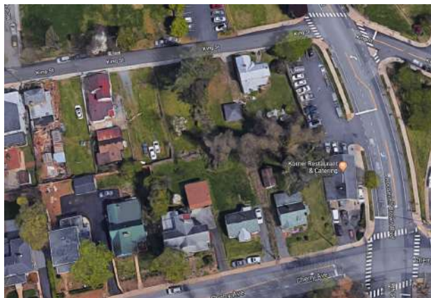
Existing aerial view of Site 10 at the corner of King Street and Roosevelt Brown Boulevard.
