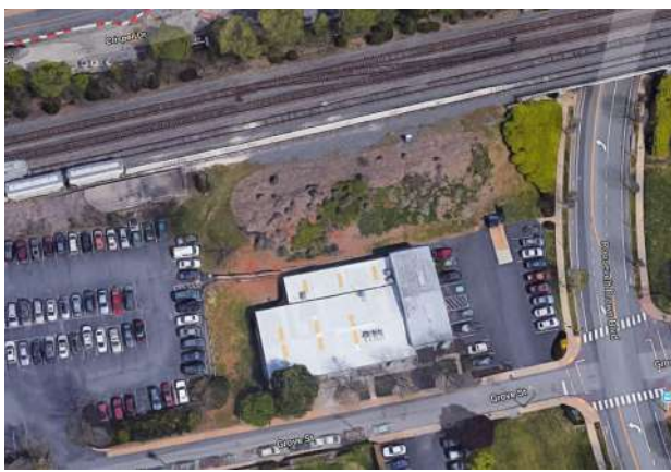
Existing aerial view of Site 12 at the corner of Grove Streets (at the bottom) and Roosevelt Brown Boulevard (to the right).
