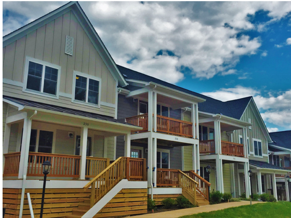
Burnett Commons - Habitat for Humanity Greater Charlottesville
